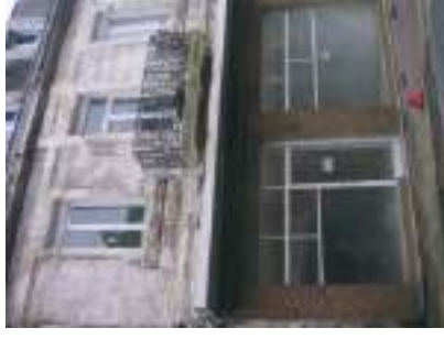
Local commercial vacant
